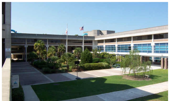
The inner courtyard of the Florida's Community College at Jacksonville, North Campus. The efficient performance of the Daikin Magnitude chiller has contributed to significant energy savings at the college, reducing the electrical usage of the North Campus during the first six months by 519,514 kWh.
