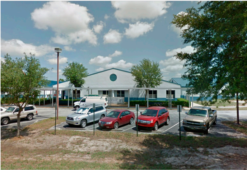
West Hernando Middle School felt effects of outdated HVAC technology chose Daikin for DOAS and VRV solutions that deliver comfort for occupants and a quick ROI for the school district.
